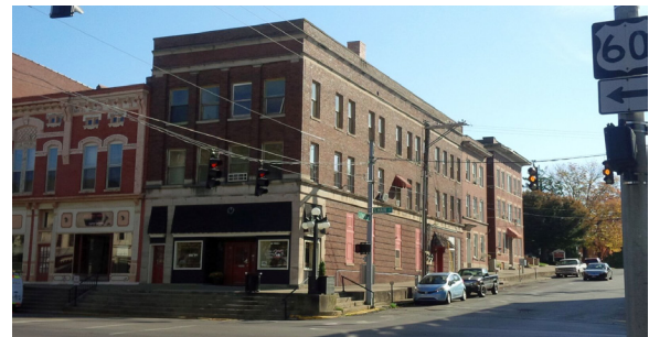
Existing Downtown Housing
